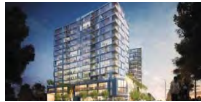
NEWSTEAD TOWER Location: Australia Total Capacity: 1,195 HP Products: CAC
